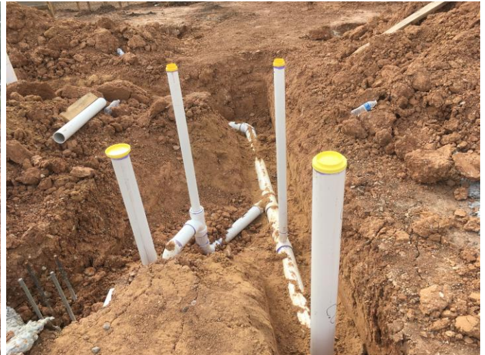
4. Underground piping for plumbing systems
