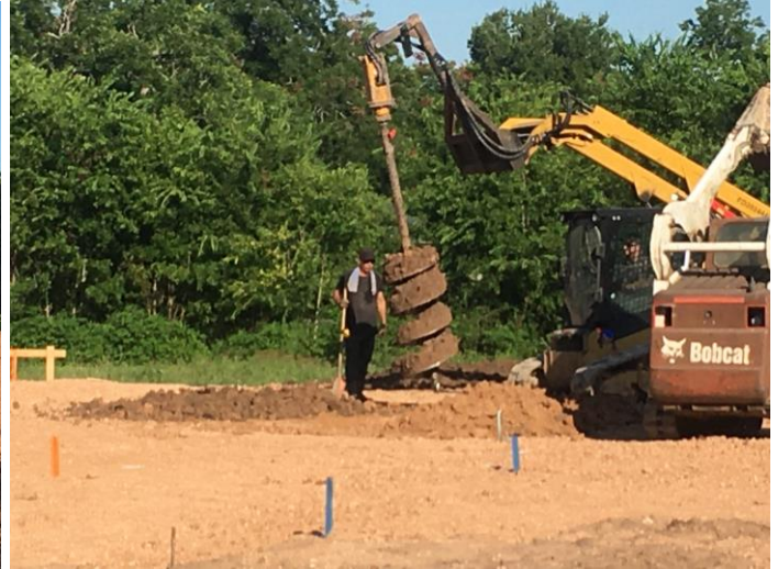
2. Equipment for drilled footing excavation
