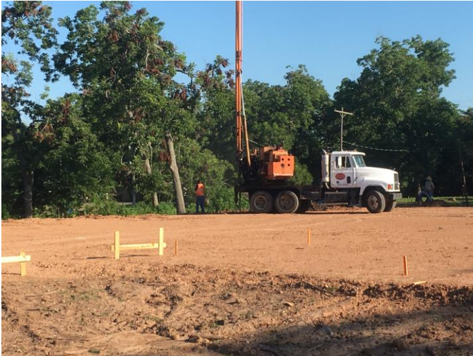
1. Equipment for drilled footing excavation
