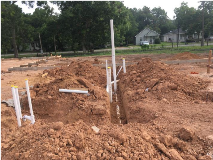
3. Underground piping for plumbing systems
