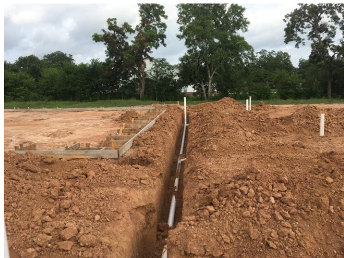
5. Concrete formwork & underground piping for plumbing systems
